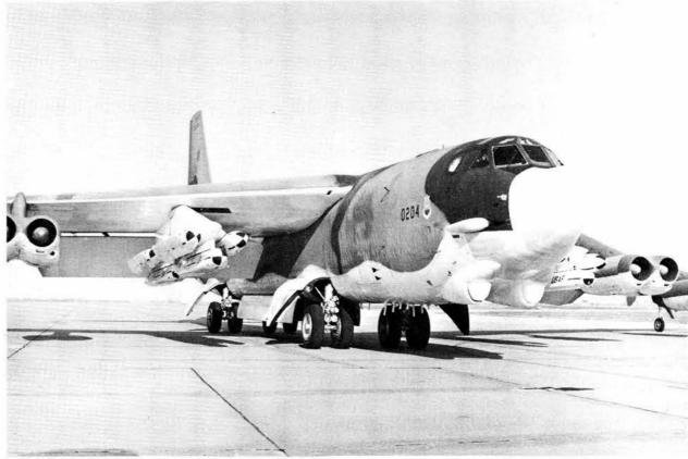
'SIX AIR LAUNCHED CRUISE MISSILES, each armed with a Sandia W80 warhead, can be mounted under each wing of the B-52 aircraft. The ALCMs can also be carrier internally in the B-52.
